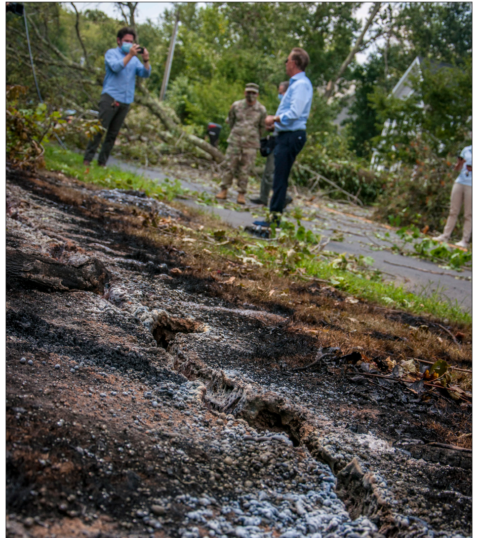
An area of scorched earth where a fallen power line caused a fire lay parallel to a road in Branford, Connecticut, Aug. 28, 2020. Maj. Gen. Francis Evon, adjutant general for the Connecticut National Guard, and Governor Ned Lamont took a tour of storm damaged towns to assess how badly the recent strong winds and tornadoes wreaked havoc in the southern region of the state.
