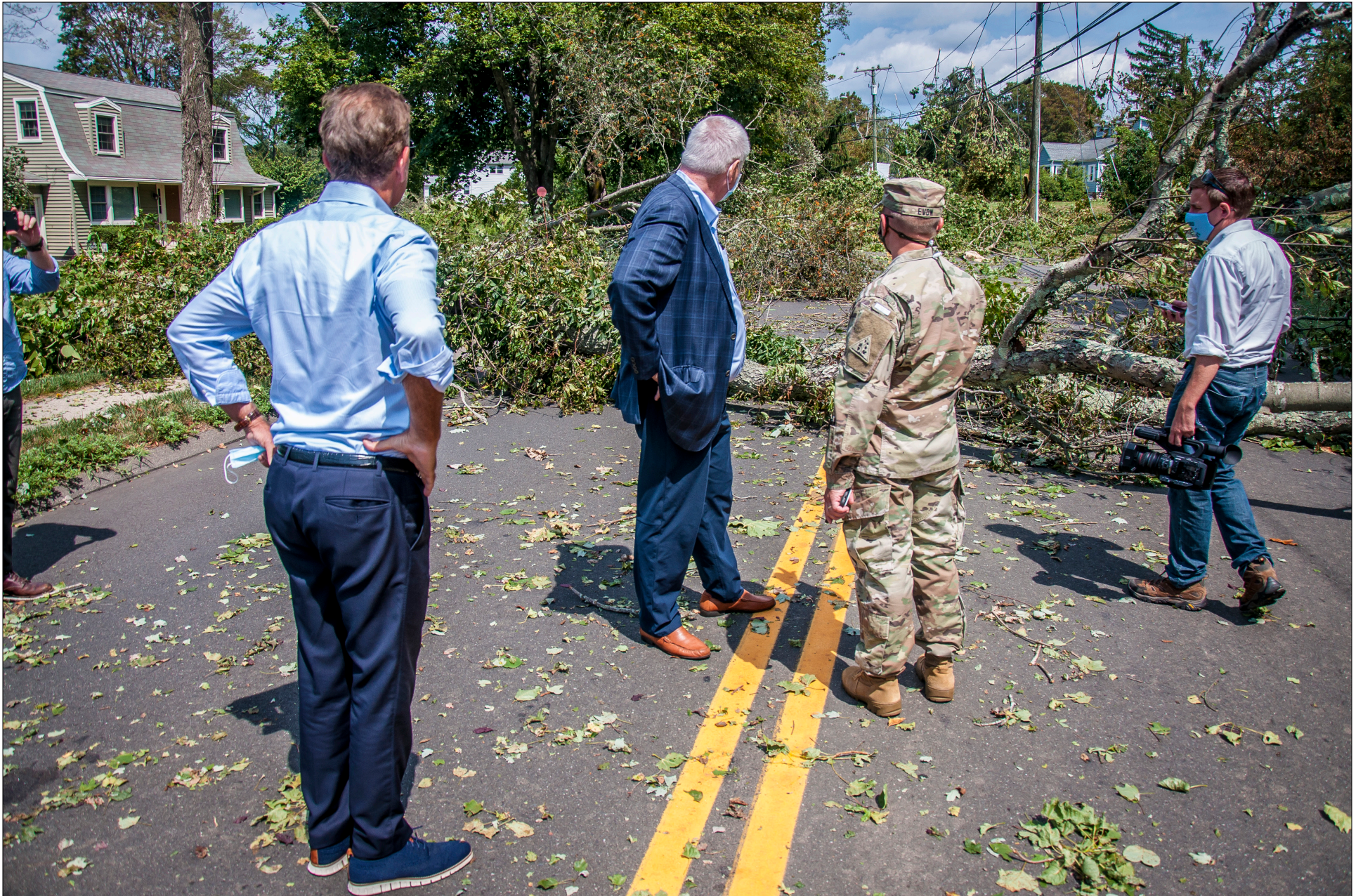
U.S. Army Maj. Gen. Francis Evon, adjutant general for the Connecticut National Guard, Governor Ned Lamont, and a representative from the local power company examine damage caused by recent storms in Branford, Connecticut, Aug. 28, 2020. Strong winds and tornadoes wreaked havoc in the southern area of the state, just days after Hurricane Isaias pummeled the region. (Photo by Tim Koster, Joint Force Headquarters Public Affairs)
